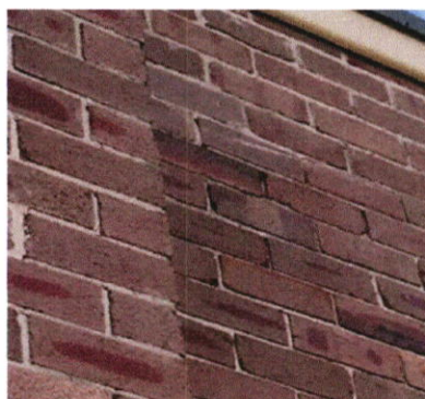
Picture of the original dwelling and extension brickwork match
